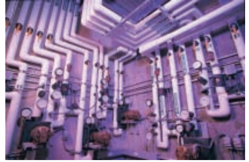
Design/Build Temperature Control System at Sonoma-Cutrer Vineyards
