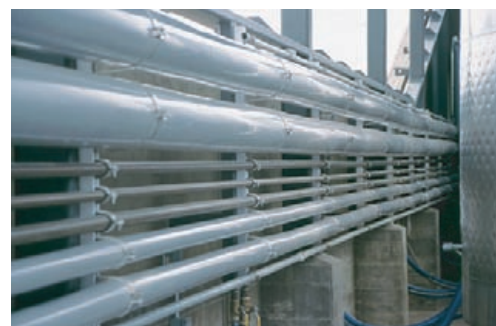
Design/Build Piping at Stryker Sonoma
